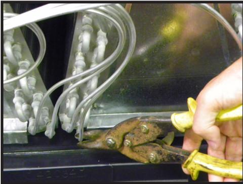
**Cut the feeder tubes where they are welded to the coil, as shown.**
